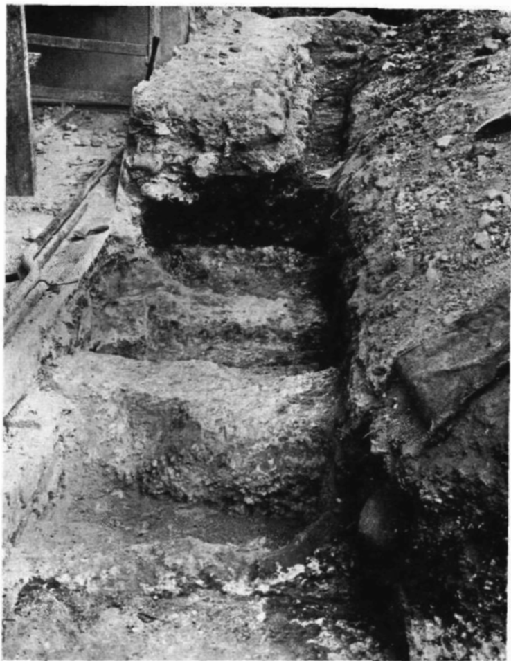
KESTON CHURCH, KENT. East wall rebuilding, 1950.
